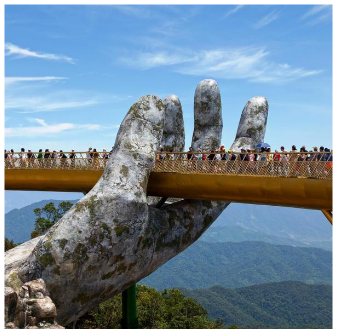
A bridge near Da Nang, Vietnam
